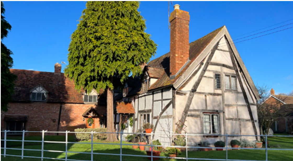
Peasant house built with crucks (large timbers extending from the ground to the apex of the roof) at Wick near Pershore, Worcestershire. A number of houses of this type in the midlands have been dated to the period 1380–1510. They were normally built by artisans (especially carpenters) employed by peasants. Image: Stephen Price
